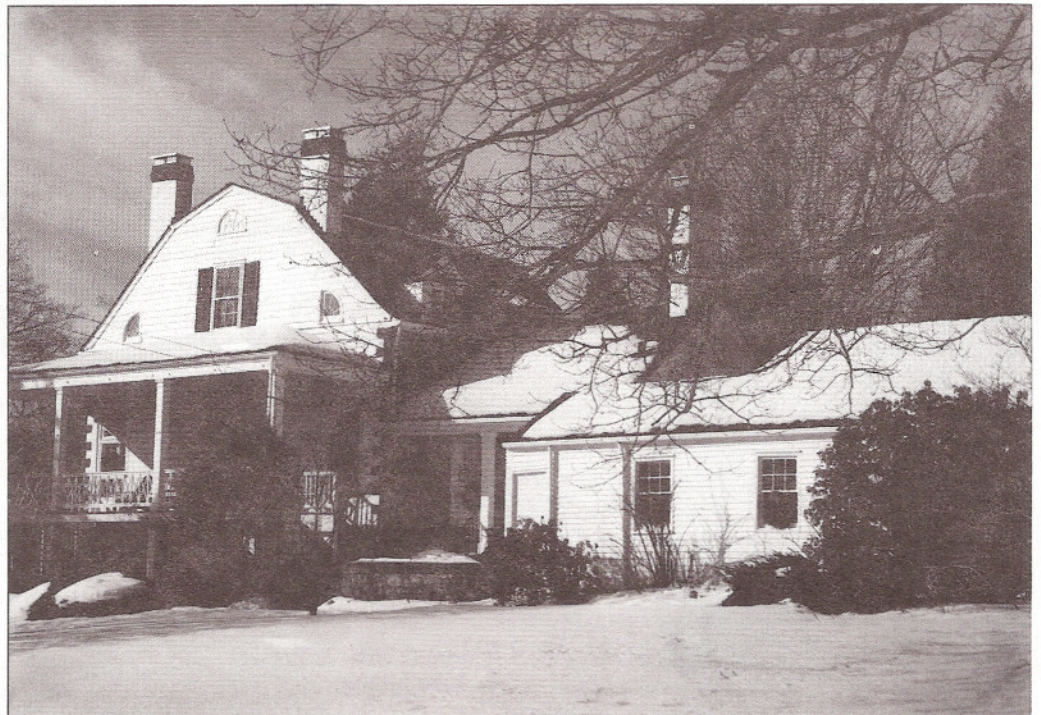
Van Voorhees-Quackenbush-Zabriskie House Photo by Marilyn Brack, 1994
